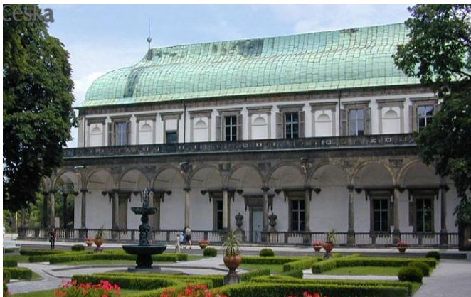
Fig. 2: Belveder roof in 2001 (before the reconstruction) [4].
